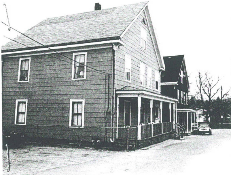
dash replaced at 41 John St., door at 3 Spruce.
